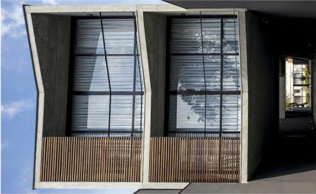
GLZ 1 ALUMINIUM FRAMED CLEAR GLAZING WINDOWS/DOORS FRAME FINISH SIM/EG TO DULUX POWDERCOAT 'MONUMENT'
