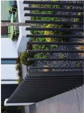
BAL 3 ALUMINIUM BATTEN BALUSTRADE SIM/EG TO KNOTWOOD 'CHARCOAL ASH'
