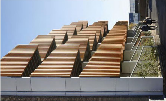
CLD 1 ALUMINIUM BATTEN CLADDING SIM/EG TO KNOTWOOD 'IROKO'
